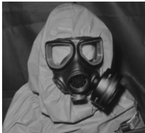
Fig. 16-6. The M17A2 Chemical-Biological Field Mask with drinking tube assembly allows the soldier to drink without unmasking. Soldiers wearing mission-oriented protective posture (MOPP) gear must drink water to prevent heat stress. The drinking tube, essentially a flexible straw, couples with the canteen cap. The soldier holds the canteen upright and inverted, then sips water through the tube. After a few sips, the soldier needs to puff his own exhaled air back into the canteen to equalize the atmospheric pressure without introducing contaminated air. Then he can take a few more sips of water before he needs to equalize the pressure again. Photograph: Courtesy of Chemical and Biological Defense Command Historical Research and Response Team, Aberdeen Proving Ground, Md.
